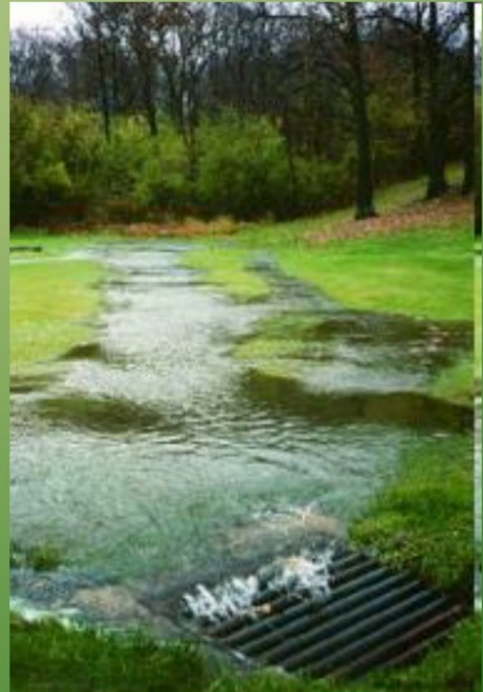
Runoff flowing into a stormwater drain
